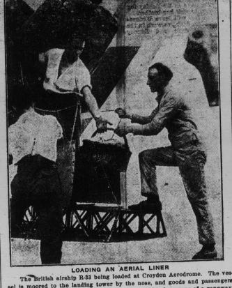
sel is moored to the landing tower by the nose, and goods and passengers are taken up through the tower and enter the airship by means of a gangway.
