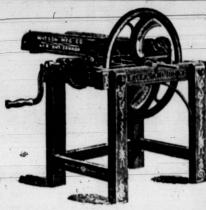
Well known and very popular all over the West. Can be operated by hand, horse, windmill or engine power. With power blower will deliver feed to any part of the barn. Will cut half a ton of hay per hour easily. Finest specially tempered English steel knives. Single lever for start, stop and reverse. Cuts ½ inch to 1¼ inch lengths by changing sprocket wheels. We make seven styles of Feed Cutters to meet all requirements. Write for FREE illustrated catalogue showing our whole line of goods.
