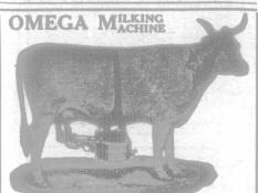
Milks fast and clean, has no rubber connections for the milk to pass through, but transparent celluloid tubes. The Omega is simple to operate, sanitary and easily washed. It is used in the private dairy of H. M. King George V. at Windsor Castle. Increased the milk flow 3%, in a 17-day test on ten cows at the O. A. C., Guelph. Write to-day for free booklet. C. RICHARDSON & CO., St. Mary's, Ont.
