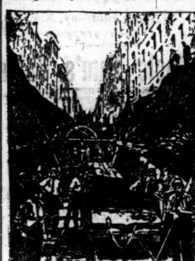
Excavating for Subway.
