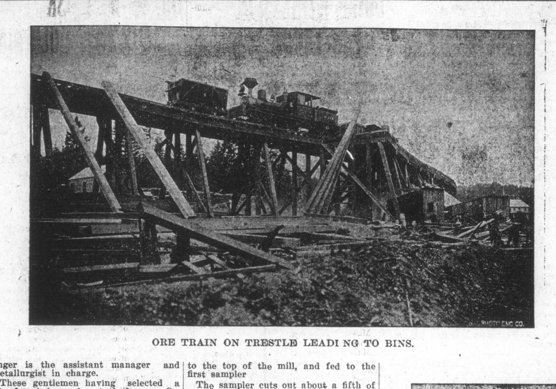
ORE TRAIN ON TRESTLE LEADING TO BINS.
