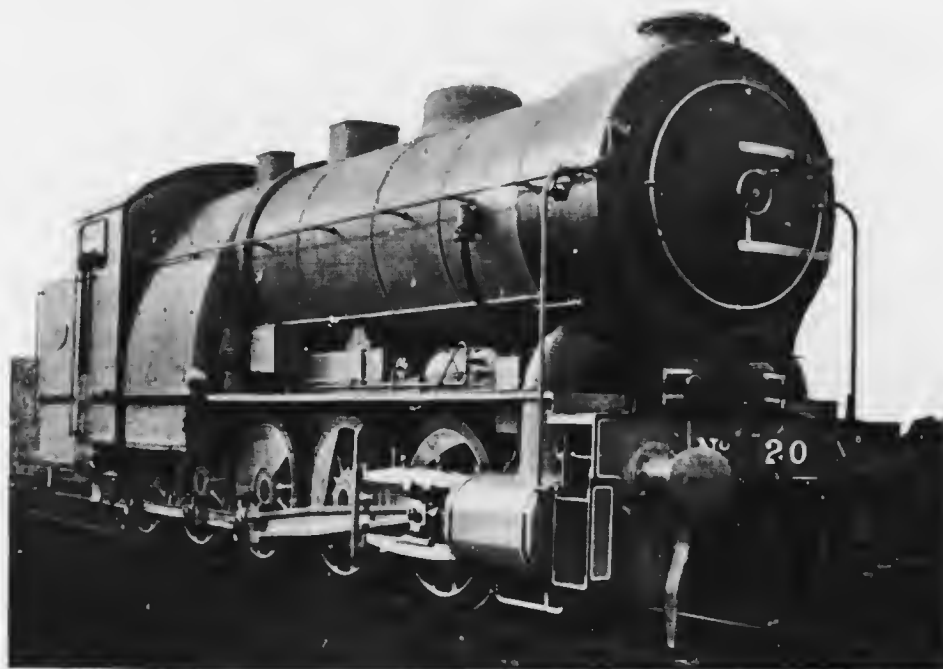
THE "DECAPOD": IT HAD FIVE PAIRS OF DRIVING WHEELS AND WEIGHED 70 TONS.
