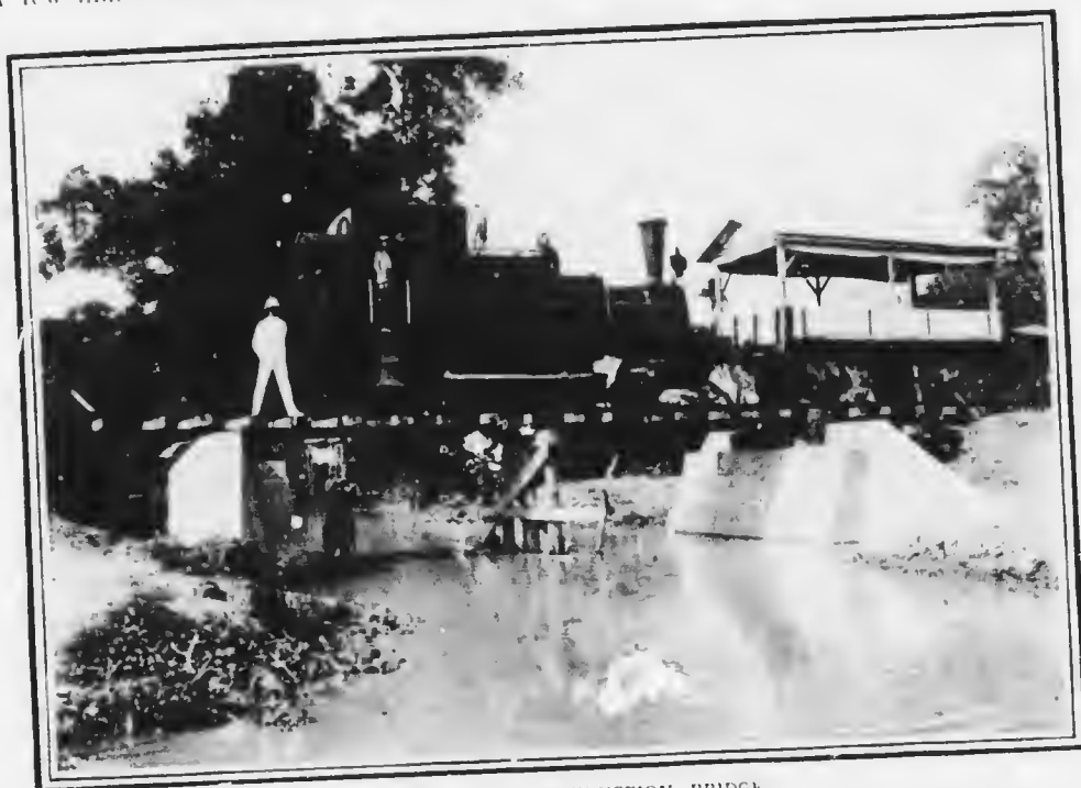
A TEMPORARY CONSTRUCTION BRIDGE.
