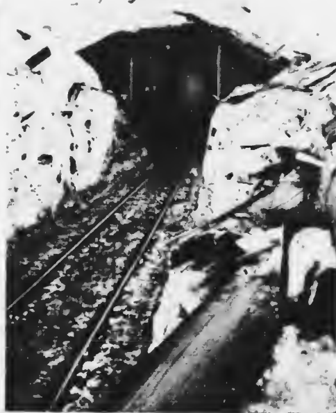
END OF SNOW-SHED AFTER SLIDE HAS BEEN CLEARED OUT.
