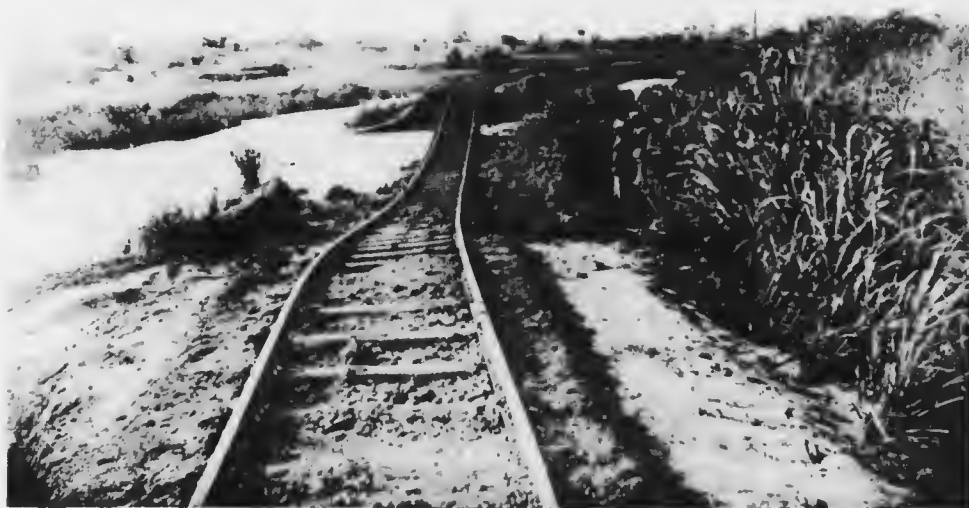
A CONSTANT MENACE TO SECTIONS OF THE GOLD COAST RAILWAY A wash-out in the Achemotah Valley.
