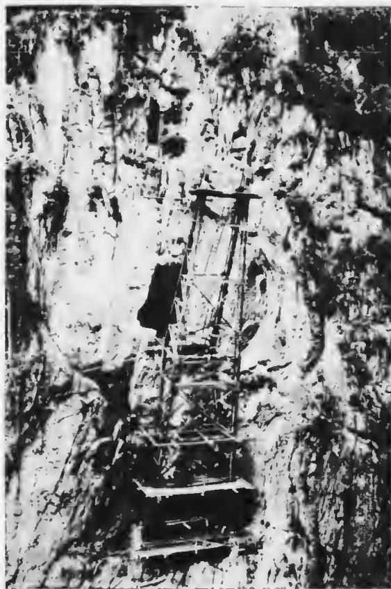
BUILDING A BASCULE OF THE FAUX NAM-TI BRIDGE UP ONE OF THE CLIFF FACES.
