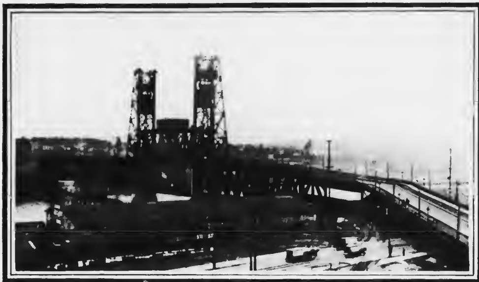
THE DOUBLE-LIFT BRIDGE AT PORTLAND OREGON
