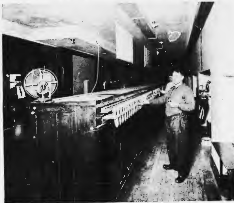
THE INTERIOR OF THE LOWER LEVEL INTERLOCKING STATION, SHOWING LEVER FRAME. This machine, 55 feet underground, contains 400 levers, and the roads which it controls cover 23 acres of ground. The lever-men merely pull the levers called out by the director.
