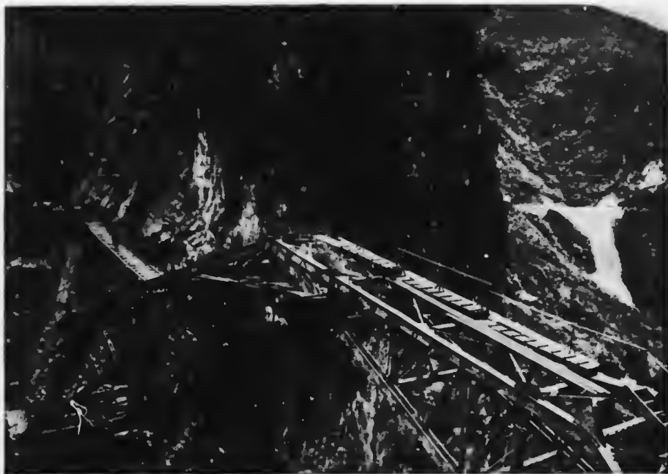
THE BASCULES OF THE FAUX NAM-TI BRIDGE, CONNECTED, SHOWING TEMPORARY GANG PLANKS.
