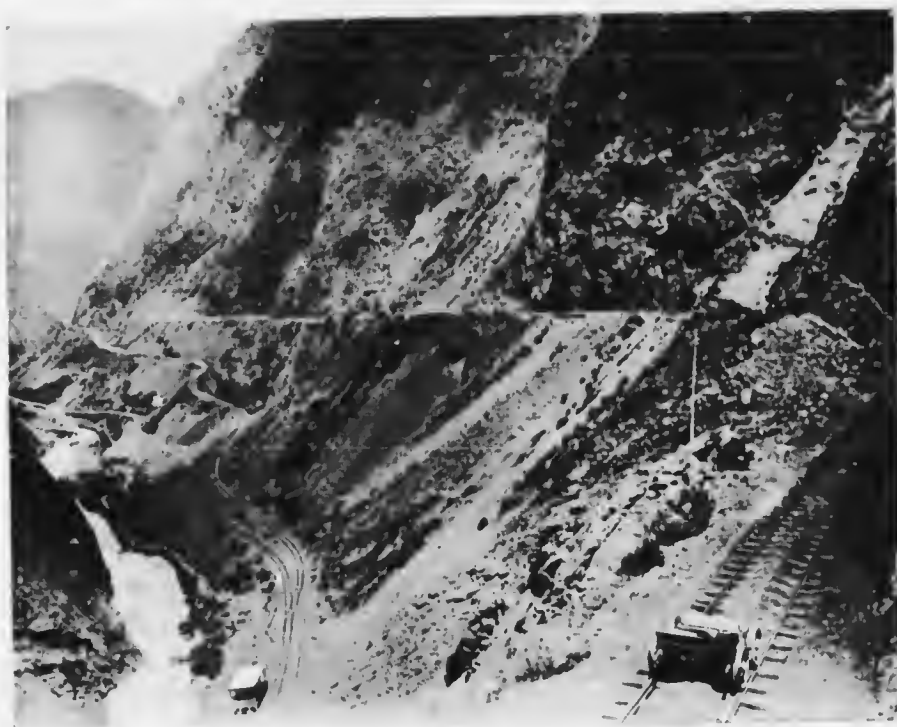
THE AMAZING TWISTS AND TURNS ON THE OROYA RAILWAY At the left is a dead end where the engine shunts to change ends of the train.
