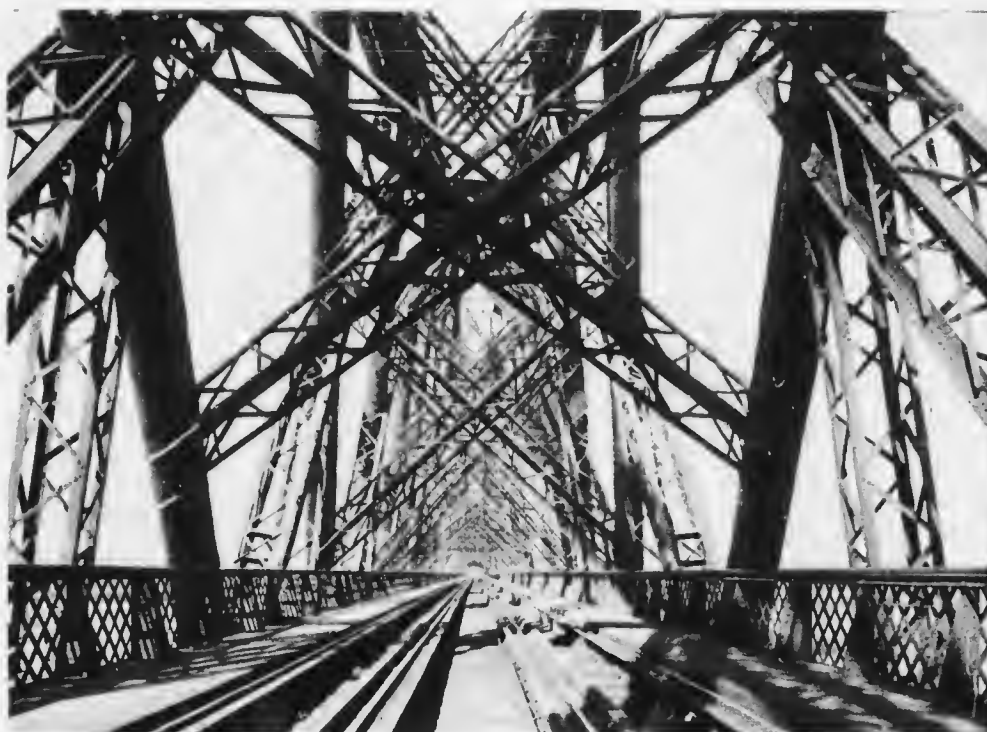
LOOKING THROUGH THE FORTH BRIDGE.
