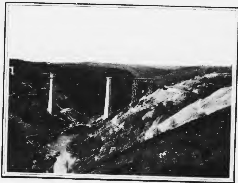
GENERAL VIEW OF THE SIOULE RIVER VALLEY AND THE VIADUCT WORKS SHOWING THE TWO CHIMNEY-LIKE PIERS
