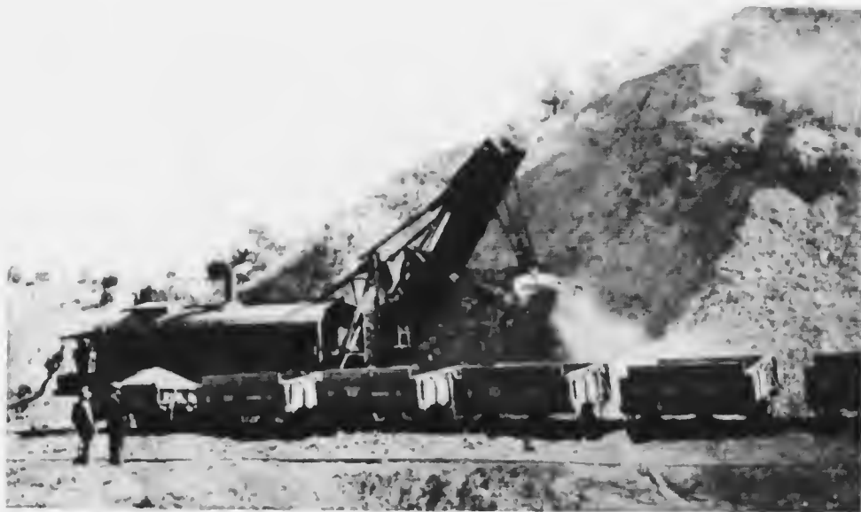
THE STEAM SHOVEL, EMPTYING ITS CAPACIOUS MOUTHFUL INTO THE BALLAST WAGONS.
