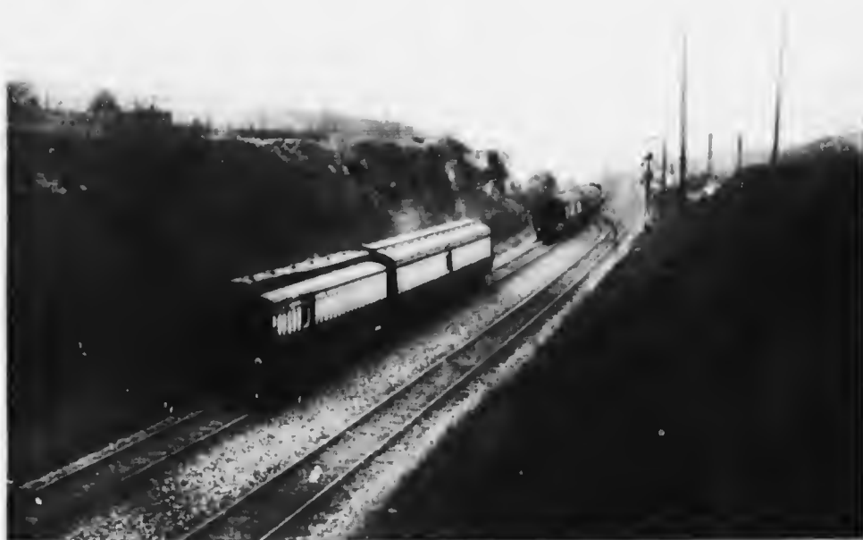
SLIPPING TWO COACHES OFF THE UP AMERICAN MAIL, WHILE TRAVELLING AT 60 MILES PER HOUR.
