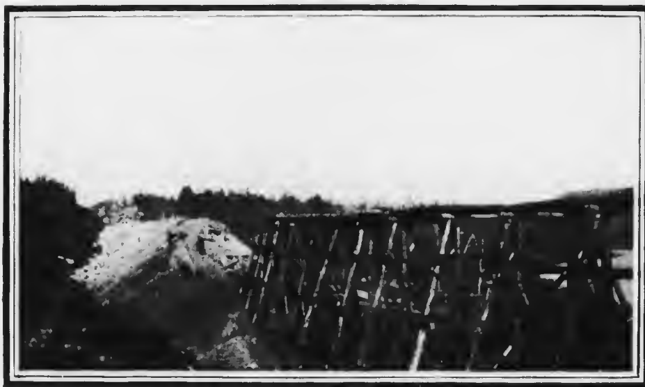
HOW THE MUSKEG WORRIES THE ENGINEER A sink in the embankment of the Grand Trunk Pacific in Quebec.
