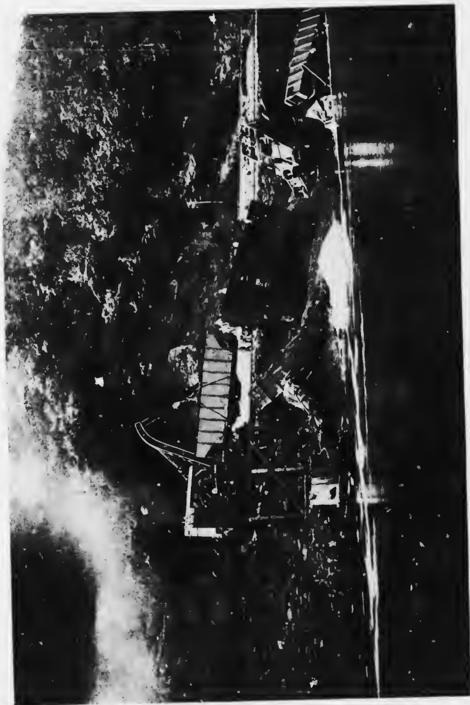
HOW THE TRACK IS CLEARED WITH FRENZIED HASTE. An Industrial Works 70-ton crane clearing the debris of a derailed mineral train. The ponderous steel cars are lifted bodily.
