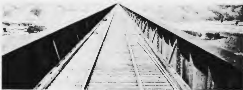
LOOKING ALONG THE DECK OF LETHBRIDGE VIADUCT Showing girders rising above the rails and forming a trough
