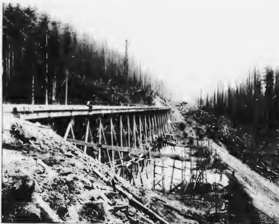
SLUICING A TRESTLE: THE LATEST METHOD OF BUILDING AN EMBANKMENT.
