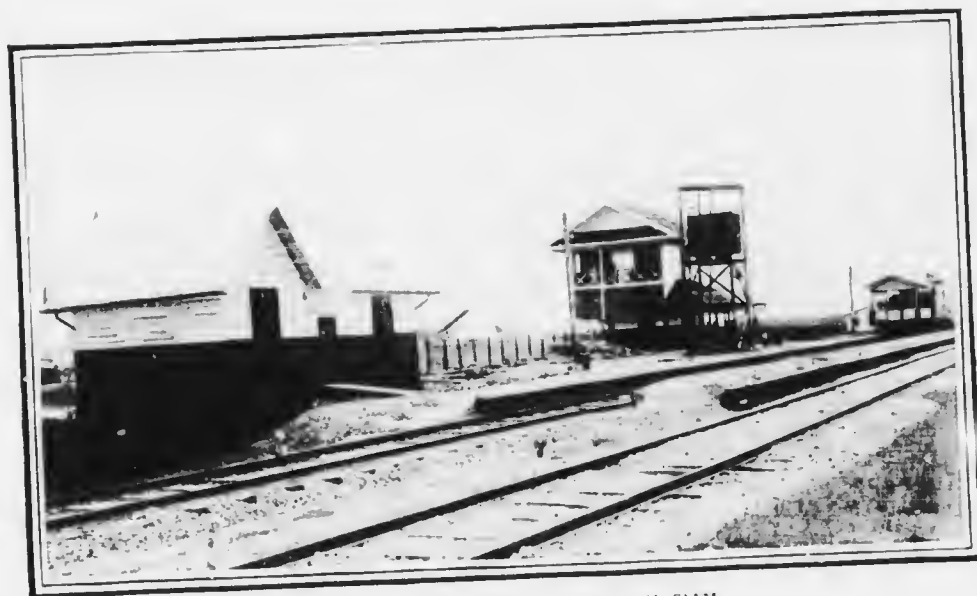
A TYPICAL UP-COUNTRY STATION IN SIAM. Showing a water tank, pumping plant and the administration buildings.
