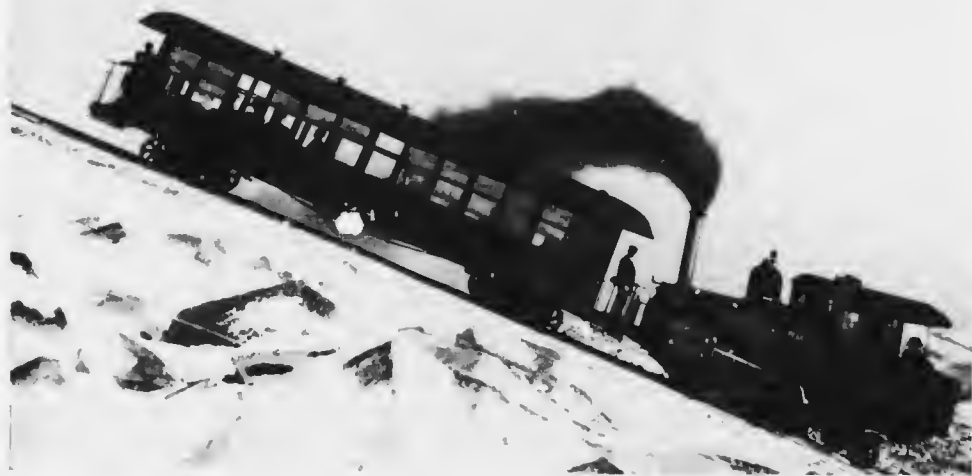
ON THE STEEPEST PART OF THE RAILWAY ABOVE THE TIMBER LINE, WHERE IT RISES 1 IN 4, SHOWING THE SPECIAL TYPE OF LOCOMOTIVE.
