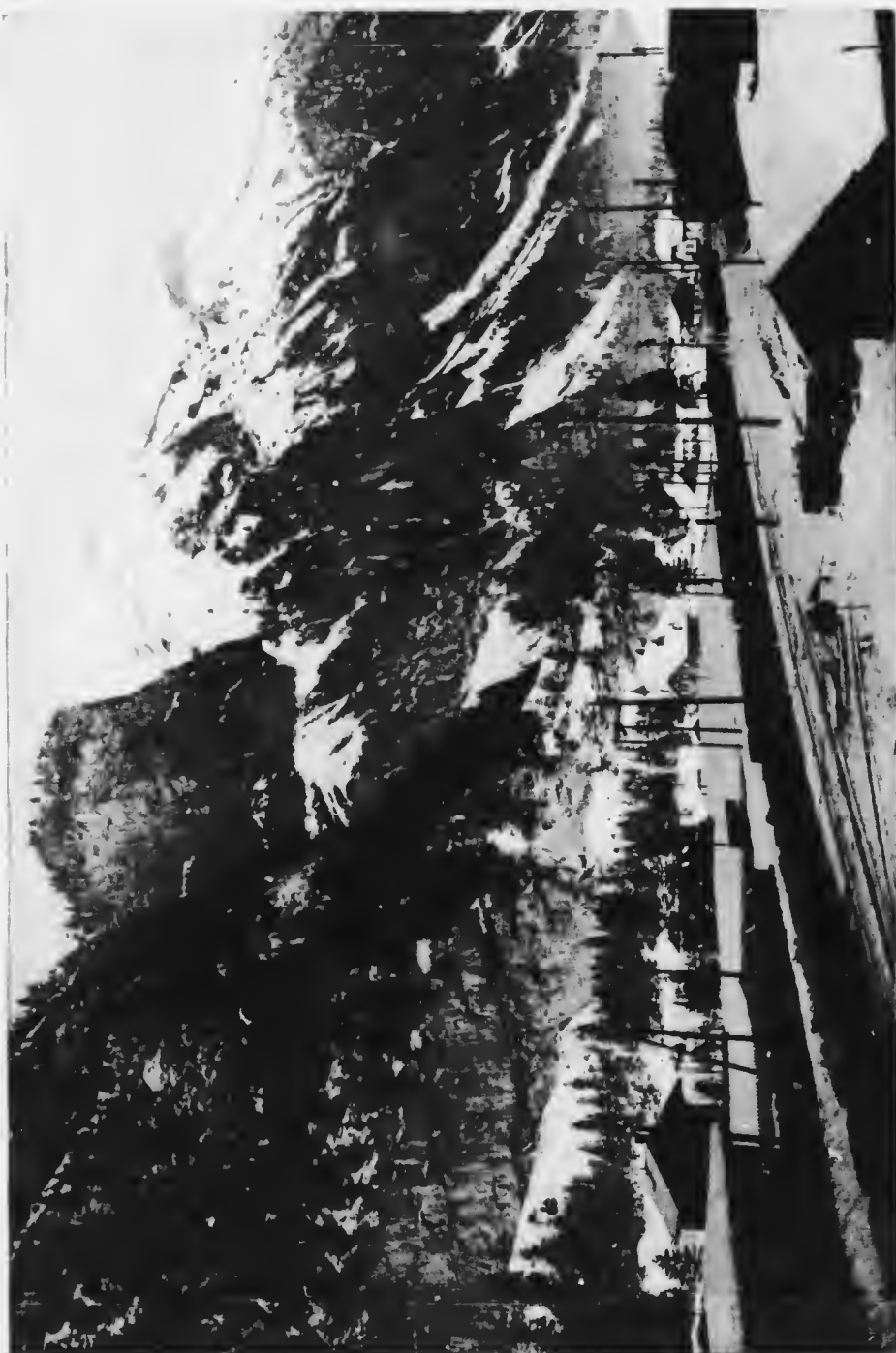
TRAIN-LOAD OF SPOIL FROM TUNNEL REPRESENTING ABOUT 3 FEET ADVANCE THROUGH THE ROCK.
