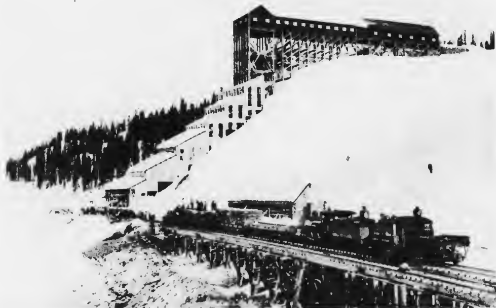
THE END OF THE TASK. LAYING THE METALS AT THE BONANZA COPPER MINE.
