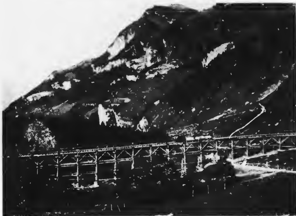
THE TEMPORARY TIMBER VIADUC*
