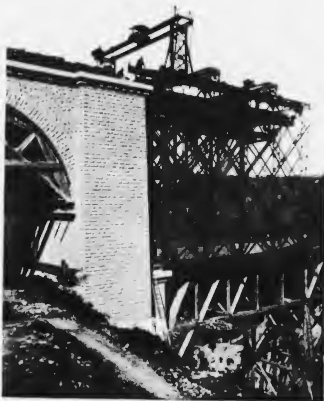
COMMENCING THE STEELWORK ON ONE OF THE SHORE SPANS SHOWING THE WIRE-NETTING ENCLOSED TRAVELLER
