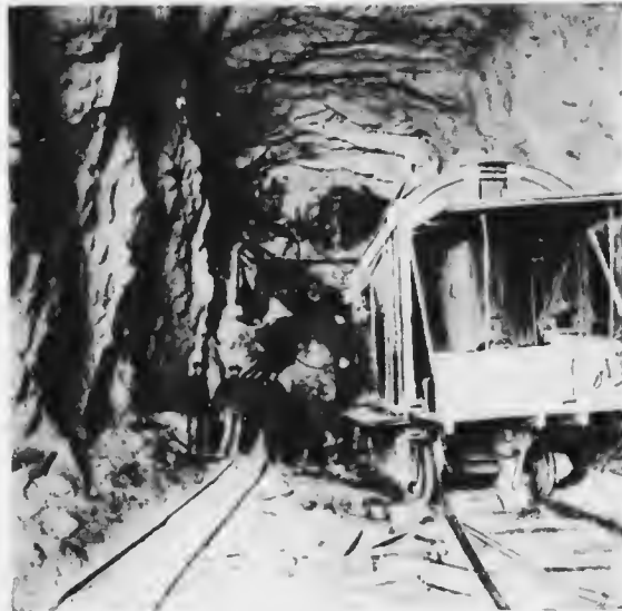
THE MECHANICAL SHOVEL WORKING IN A TUNNEL AND DRIVEN BY COMPRESSED AIR.
