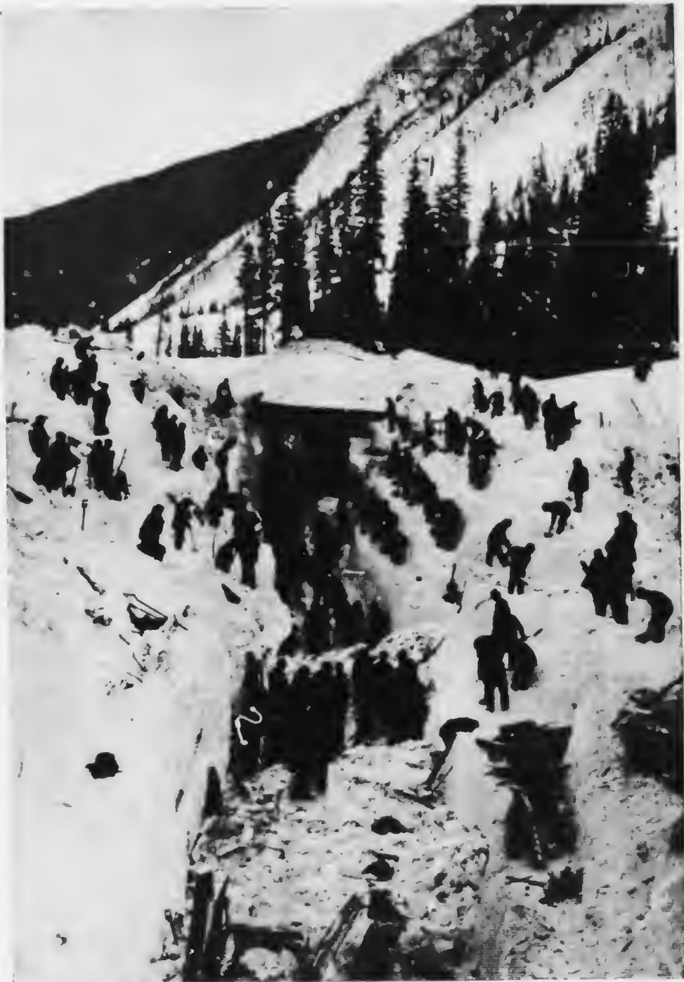
CLEARING A SLIDE FROM THE TRACK BY HAND.
