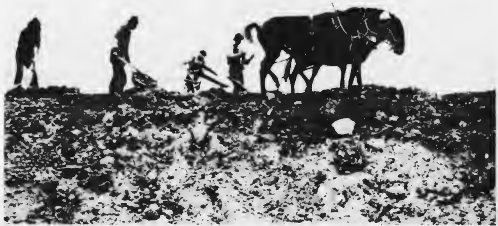
PLOUGHING OFF THE TOP OF A HILL TO LEVEL THE GRADE ON THE CANADIAN NORTHERN TRANSCONTINENTAL.
