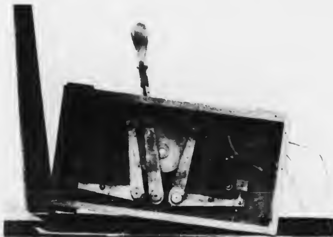
THE CONTROLLER OF EDISON'S FIRST ELECTRIC LOCOMOTIVE.
