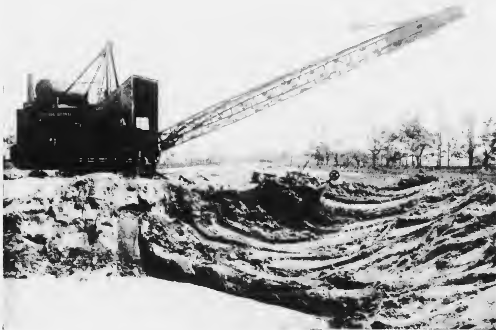
Photograph by permission of the Bucyrus Company. DRAG-LINE EXCAVATOR WORKING IN HEAVY CLAY IN A BALLAST PIT Showing how the ground is scooped out.
