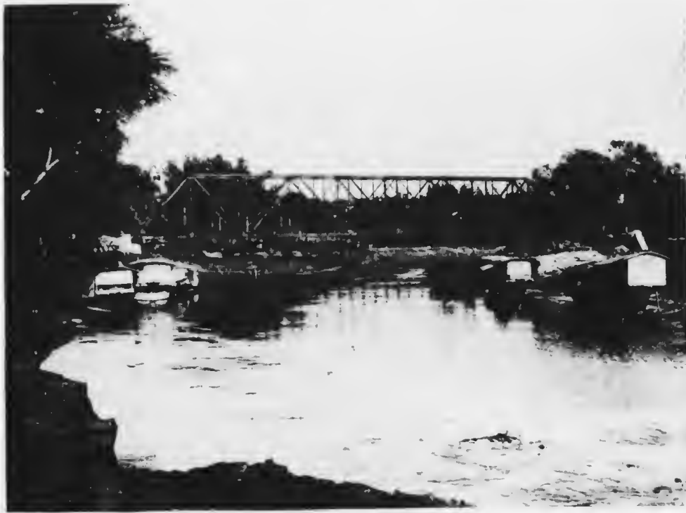
A SINGLE SPAN BRIDGE OVER THE KLONG THIA LAW, ON THE NORTHERN RAILWAY, SIAM. The span is 263 feet. On the river are some of the quaint craft by which transportation was effected before the railway was built.
