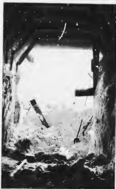
SNOW-SLIDE SCENE AT ROGERS POINT. Looking out of snow-shed partly covered by slide.
