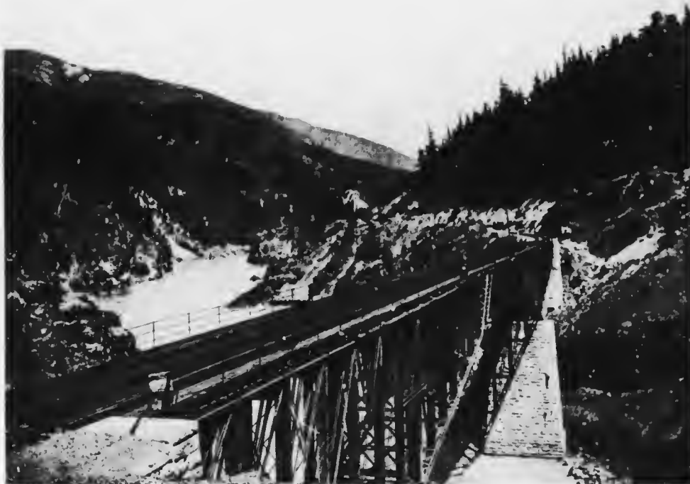
THE BRIDGE OVER FRASER CANYON.
