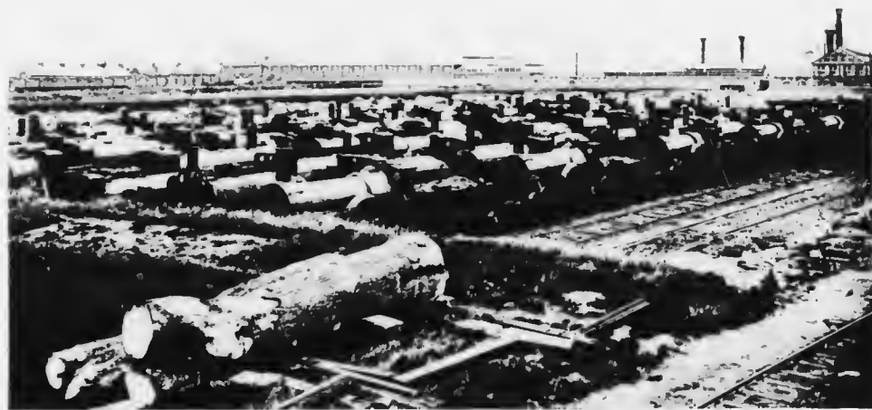
A LOCOMOTIVE GRAVEYARD BROAD GAUGE ENGINES AT SWINDON STATION, MAY, 1892. Withdrawn from service by the conversion of the gauge from 6 feet to 4 feet 8½ inches.
