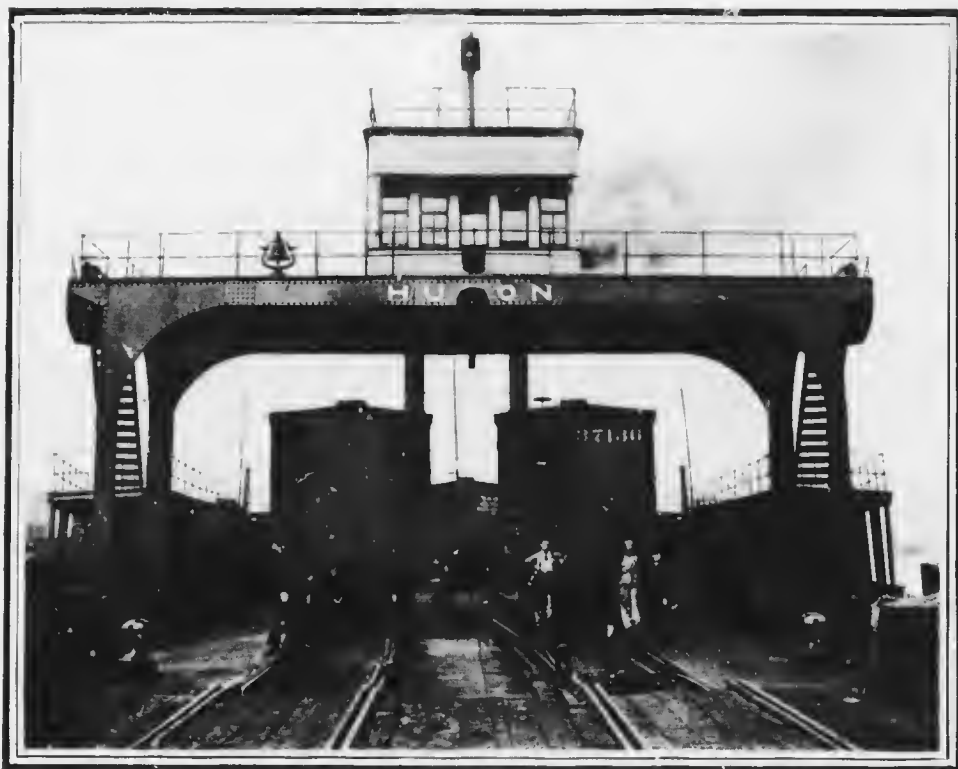
THE TRAIN DECK OF THE HURON , WHICH PLIES ACROSS THE DETROIT RIVER BETWEEN WINDSOR AND DETROIT.
