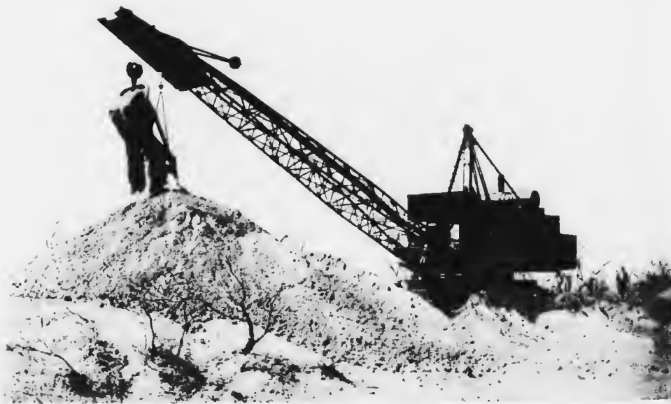
THE DRAG-LINE EXCAVATOR BUILDING UP AN EMBANKMENT
