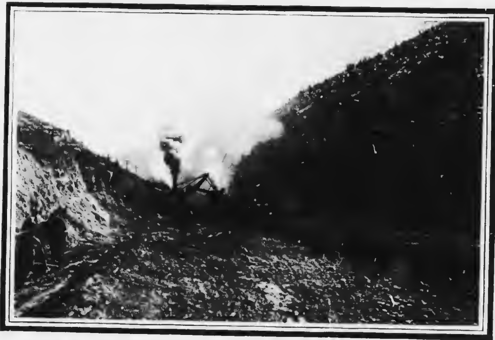
CUTTING OUT THE SOLDIER SUMMIT HUMP ON THE DENVER AND RIO GRANDE RAILWAY. By this work a rise of 105, instead of 211 feet, per mile is secured.
