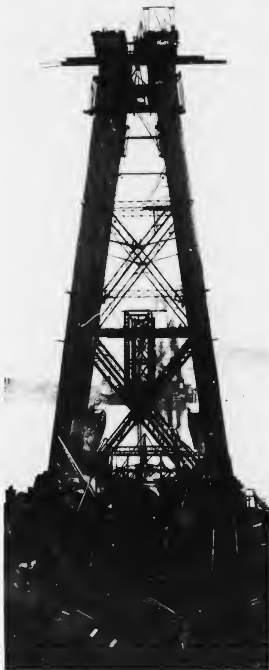
RAISING THE MASSIVE STEEL LEGS ON THE FIFE PIER, APRIL 15, 1887.
