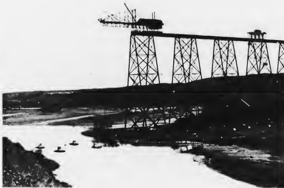
BUILDING THE LETHBRIDGE VIADUCT
