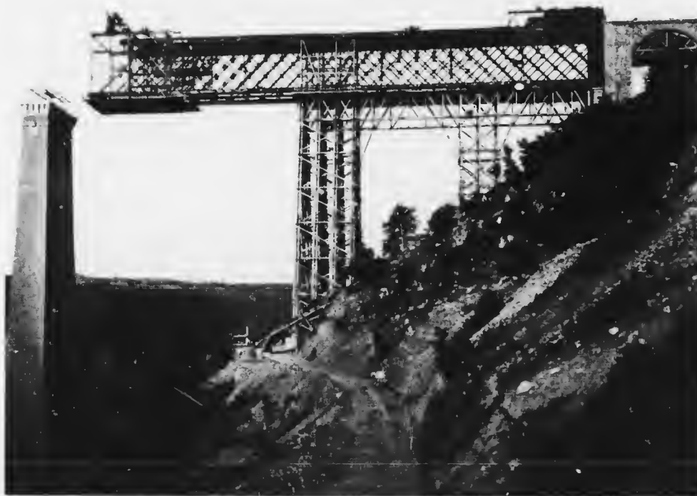
CRAWLING FOOT BY FOOT TOWARDS THE FIRST PIER.
