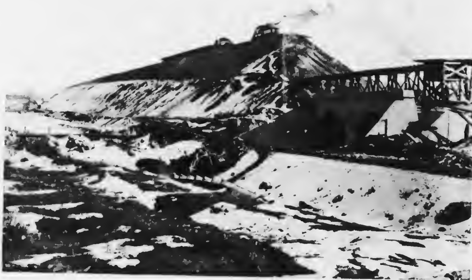
BUILDING UP THE PEQUEST FILL ON THE LACKAWANNA CUT OFF This enormous embankment absorbed over 6,600,000 cubic yards of material.
