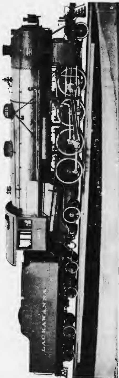
A DELAWARE, LACKAWANNA AND WESTERN RAILROAD MAMMOTH. Its weight in working order, with loaded tender, is 235.85 tons.
