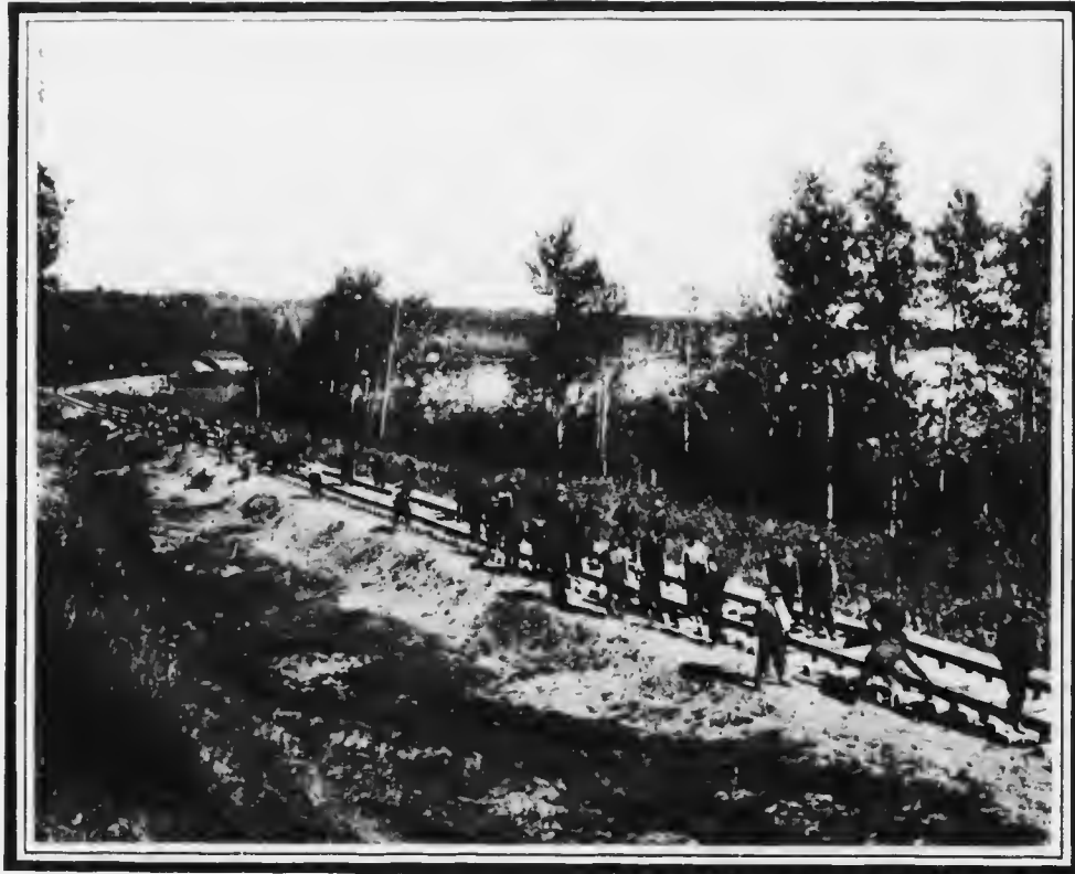
The photograph is by permission of the General Land Office, U.S. Forest Service. THE "LIFTING" GANG TRUE-ING, LIFTING AND LEVELLING RAILS AND COMPLETING SPIKING TO SLEEPERS.
