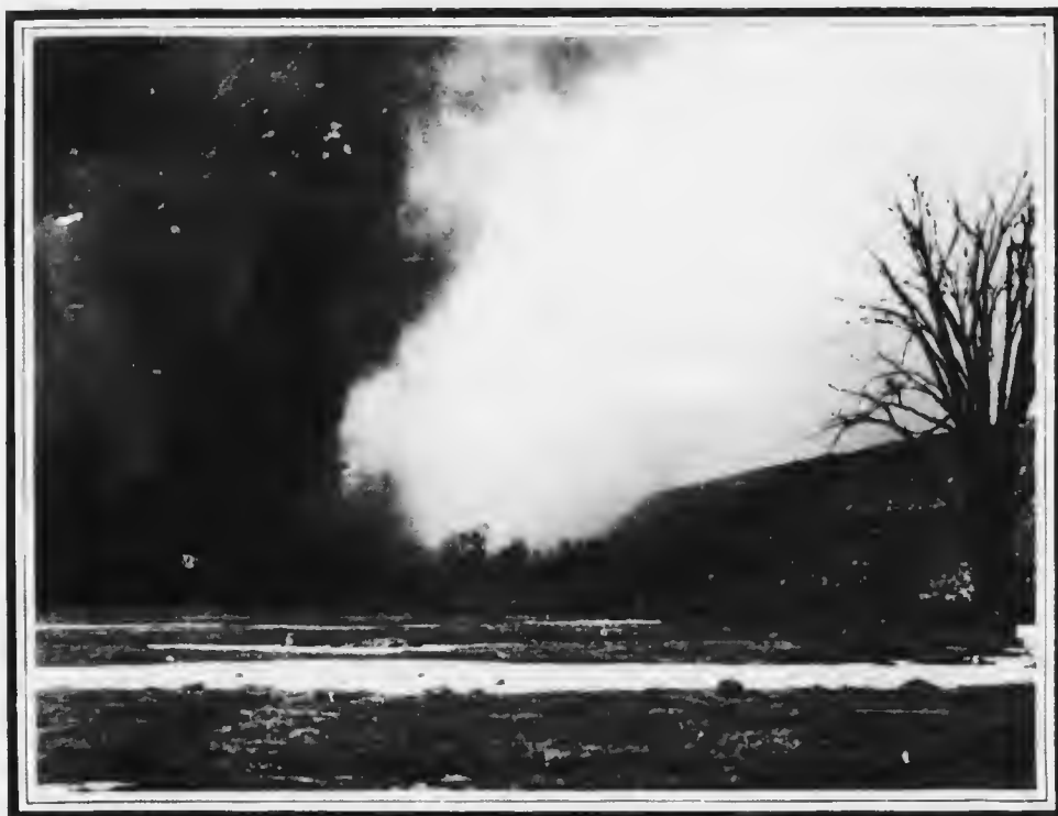
A 16½ TON BLAST ON THE LACKAWANNA CUT OFF. 5,000,000 lb. of dynamite were used in this reconstruction work.
