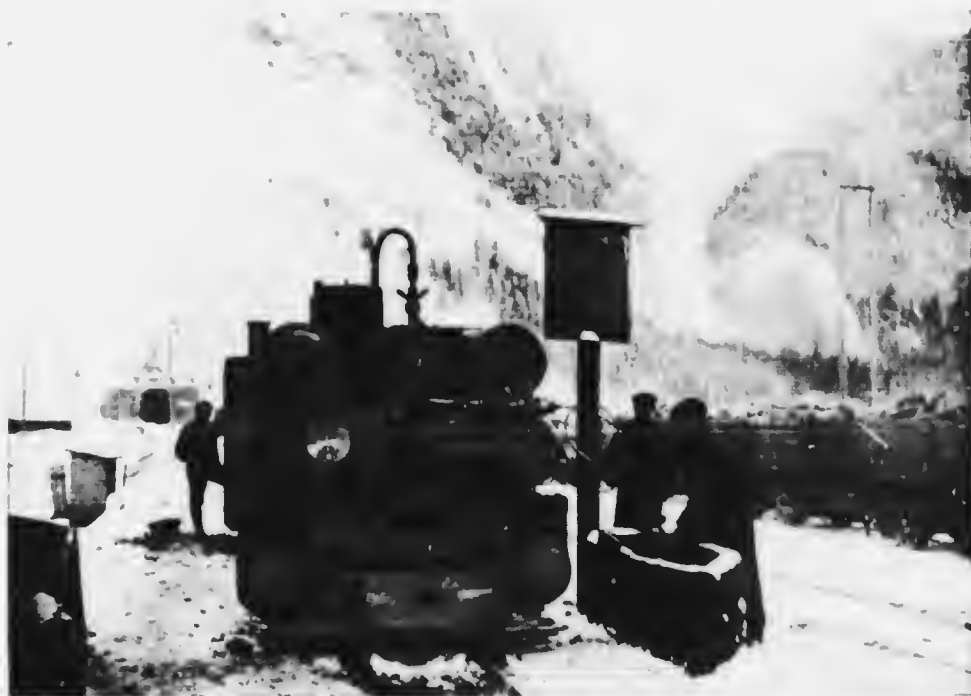
CHARGING A COMPRESSED-AIR ENGINE AT KANDERSTEG.
