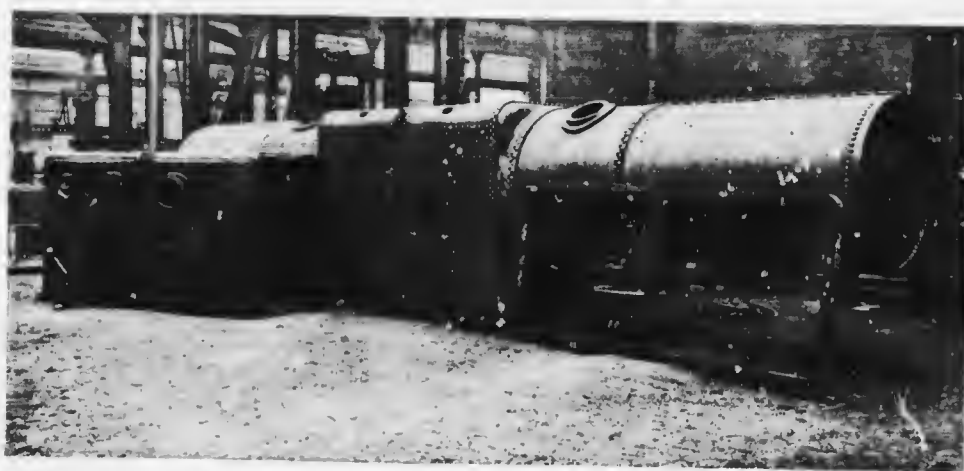
THE DOUBLE BOILER, FIRE-BOXES, AND FOUNDATION RING OF THE LARGE "FAIRLIE" ENGINE BUILT FOR THE MEXICAN RAILWAY
