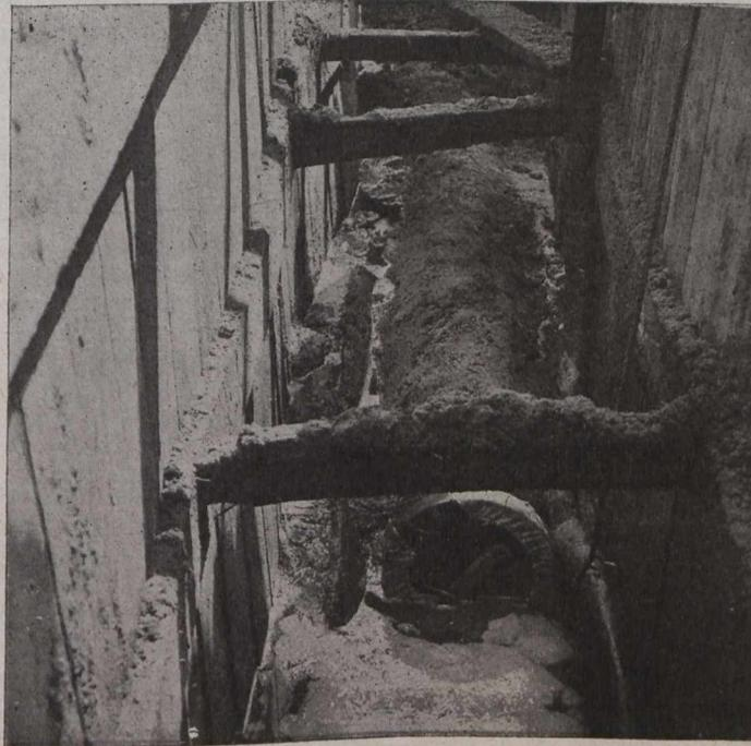
Fig. 1.—Showing Canvas Cover in place on bell end of pipe, ready for spigot end of next pipe. This view shows the efficiency of these covers. Note the water in the trench, kept out of pipe by the covers over the joints in background, which are concealed under 3 inches of concrete.
