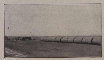
Fig. 2.-Steel Forms for Circular Pipe.
