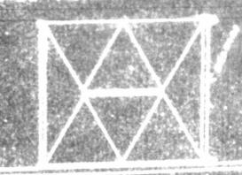
After the experiment with the Ring-Rite, July 7, 1908, noted in Bulletin No. 1, the kite was strengthened by beading connecting the lower and upper aeroplanes. To offest this additional weight the inner rings of beading on the two aeroplanes were removed, with the net result that the kite was lighter as well as stronger than before. For details of construction see Mr. Bedwin's article in this Bul-letin.
