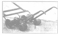
This Seeder is made both single and double, and in either form is without an equal as a compact handy implement. The seed-box is run by a friction gear, and can be stopped and started instantly without stopping the horse. It can be regulated to sow any desired quantity of turnip, mangold or carrot seed.
