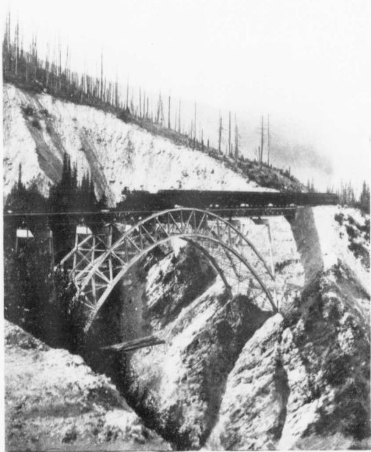
STONY CREEK BRIDGE, BRITISH COLUMBIA.
