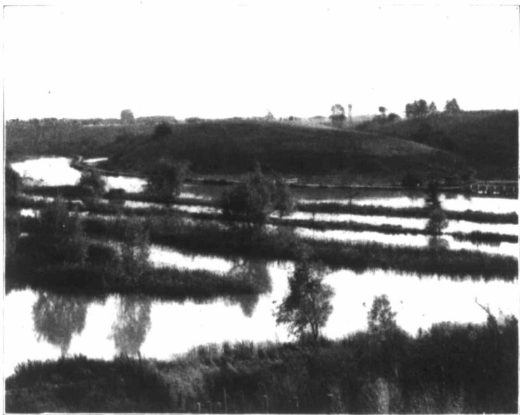
ABOVE LOCK 2, OLD CANAL.
