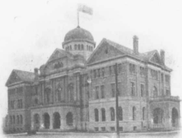
COURT HOUSE AS REBUILT 1899.
