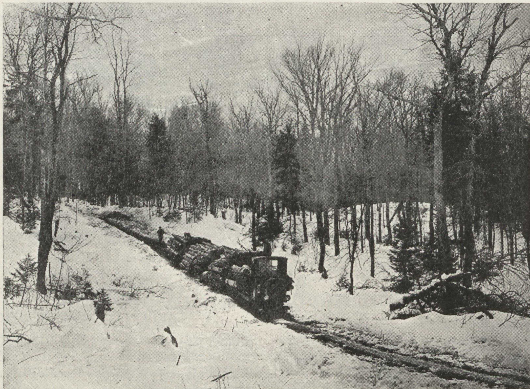
Tractor and Train at foot of 35 p.c. down grade
