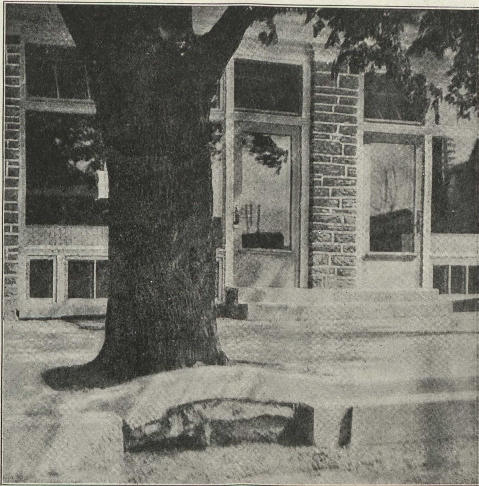
AN UNUSUAL AND EFFECTIVE CURB TREATMENT
