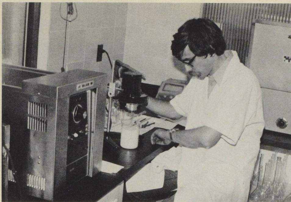
Development of a fortified skim milk sterilized by the ultra high temperature system with added milk proteins and vitamins, has been completed. Lester Dobosz measures the viscosity of the finished product. (Photo: Nelson's Dairy)
