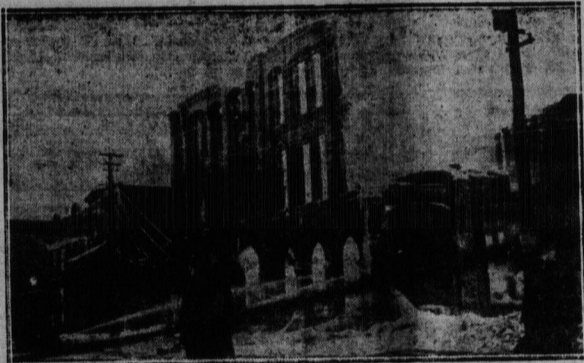
THE FRONT OF BUILDING AFTER THE FIRE
