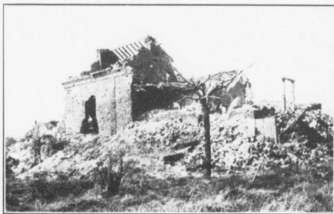
BATTERY OFFICE, ST. PIERRE.
