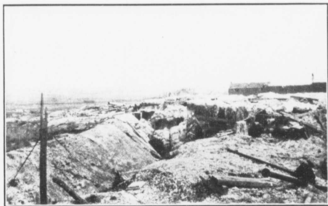
LOOKING DOWN TRENCH IN REAR OF GUNS—LIEVIN.
