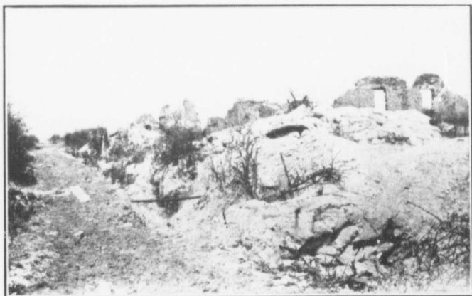
BATTERY POSITION, CITE ST. PIERRE.
