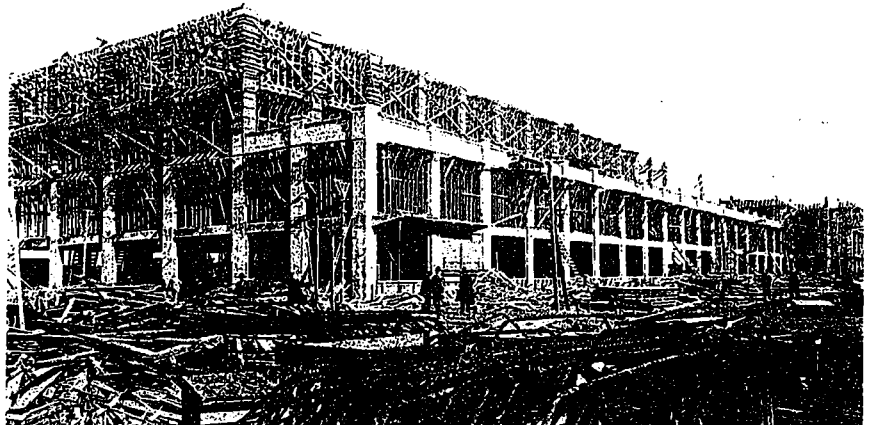
LOOKING NORTH-EAST, BUILDING NO. 3, NOVEMBER 4TH, 1914.
