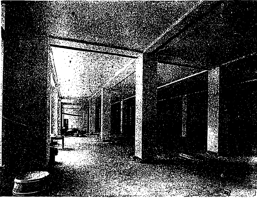
CHRISTIE, BROWN & CO., LTD., BUILDING, OFFICE BEFORE SCREENS WERE INSTALLED. (DARK LINES ON BEAMS AS BRICKS FOR SCREENS).
