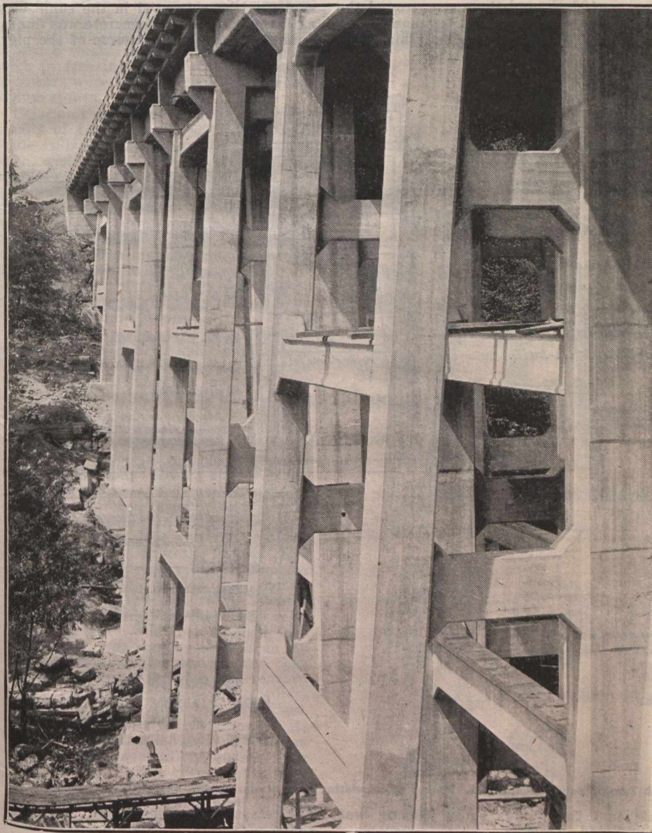
Bridge over Reservoir Park Ravine, North Toronto Subdivision, C.P.R.
