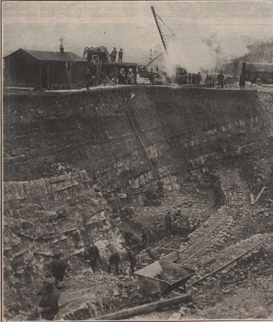
Canadian engineers working a quarry for road making material, on the Western Front. Canadian Official War Photograph. Copyright reserved.
