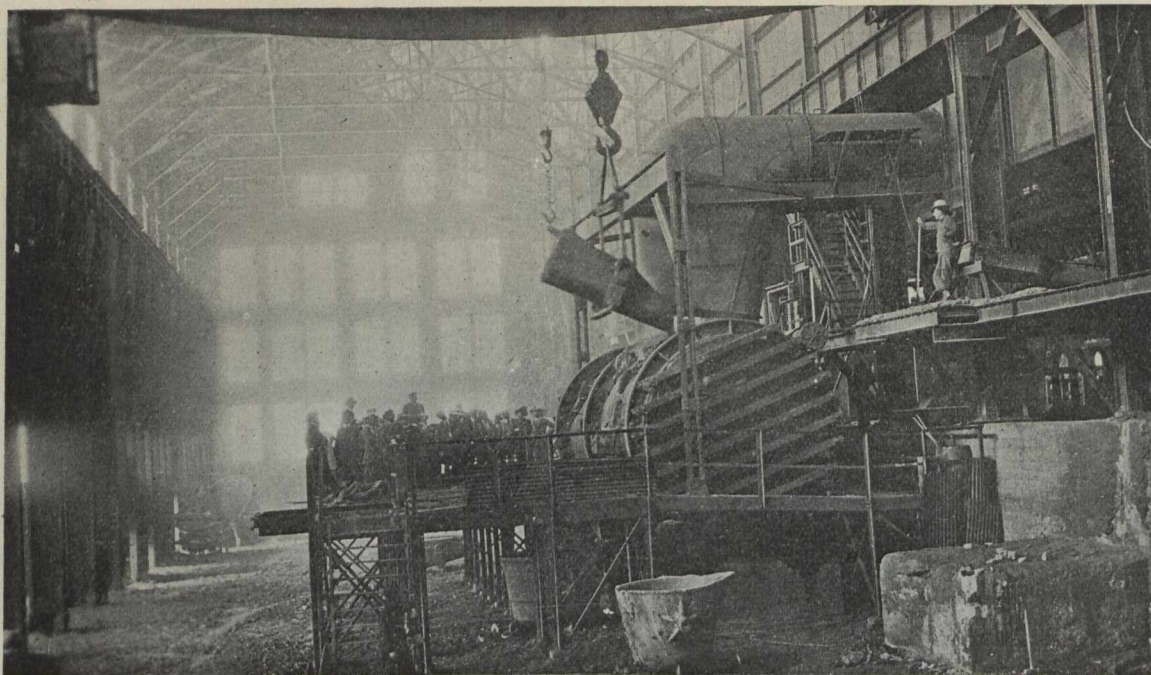
Charging a basic converter, at new smelter of Mond Nickel Co., at Coniston, Ont.
