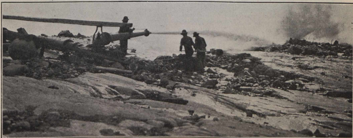
Washing rock surface to expose veins, Nipissing mine, Cobalt
