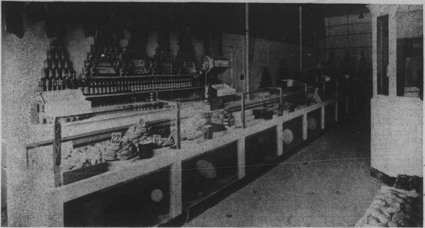
View of the refrigerator counters in the Wm. Rowntree & Son store, Dundas Street, Toronto. These counters are on three sides of the store.
