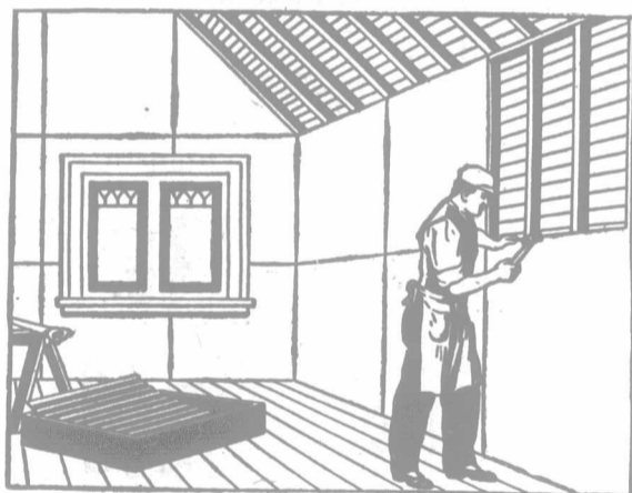
Applying Wall Board to Studding
