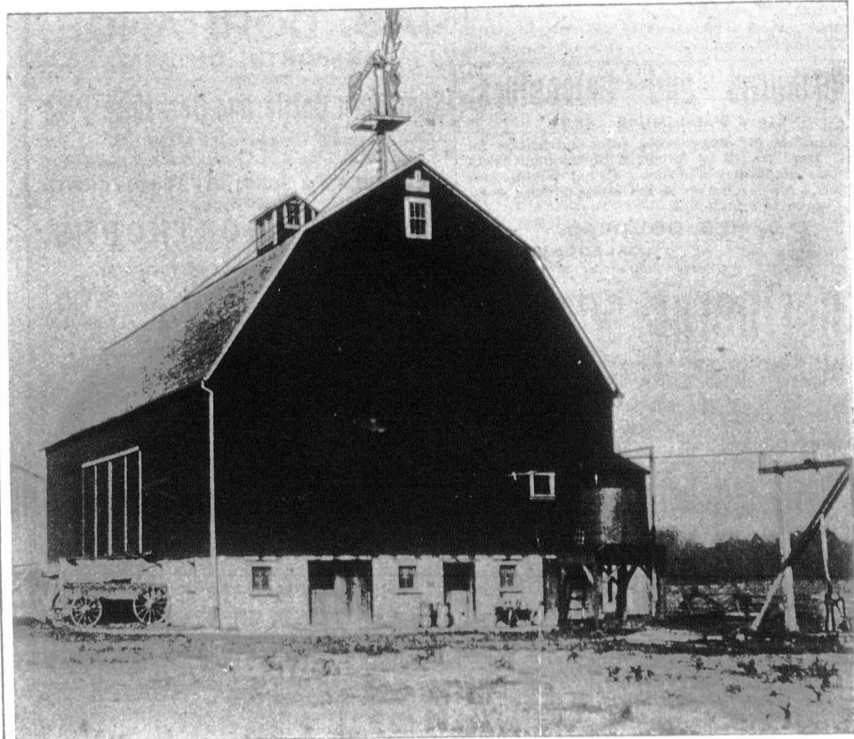
Stock barn of Mr. John D. Ferguson, in the township of Yarmouth. Dimensions of the building, 80 x 48 feet; foundations of concrete, 2 1/2 feet deep. Floors and root cellar all of Thorold Cement.
