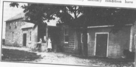
An Up-to-date Cheese Factory in Peterboro Co., Ont. owned and operated by R. H. Little. This factory is made of hollow cement blocks. Most of the work of construction was done by Mr. Little. To the left can be kept clean with a minimum amount of work. Mr. Little and his son are
