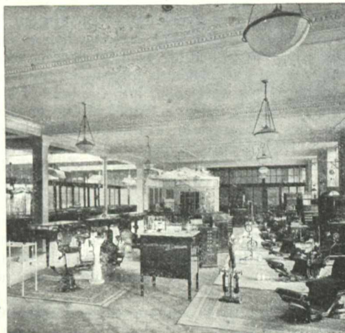
Section of The D. M. Co.'s London Showroom, Alston House, Newman Street, London, W.
