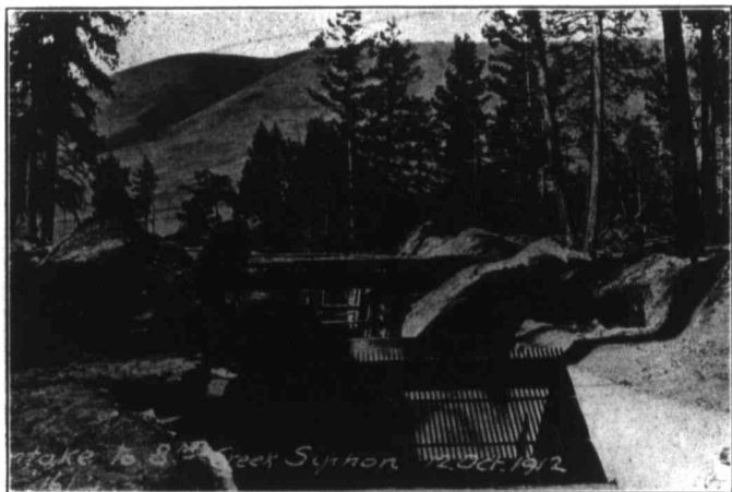
Fig. 5.—Intake to 8-Mile-Creek Siphon.
