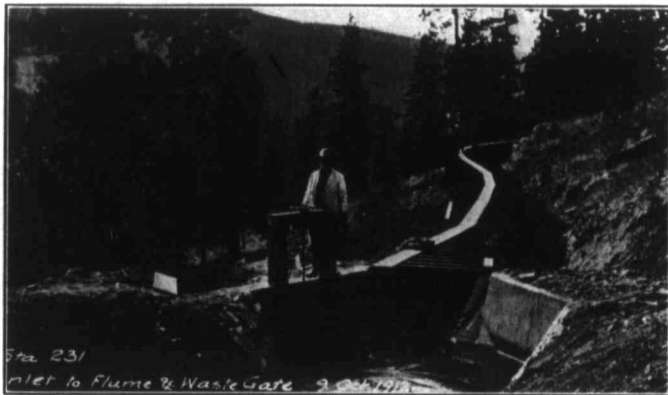
Fig. 4.—Inlet to Flume and Waste Gate.
