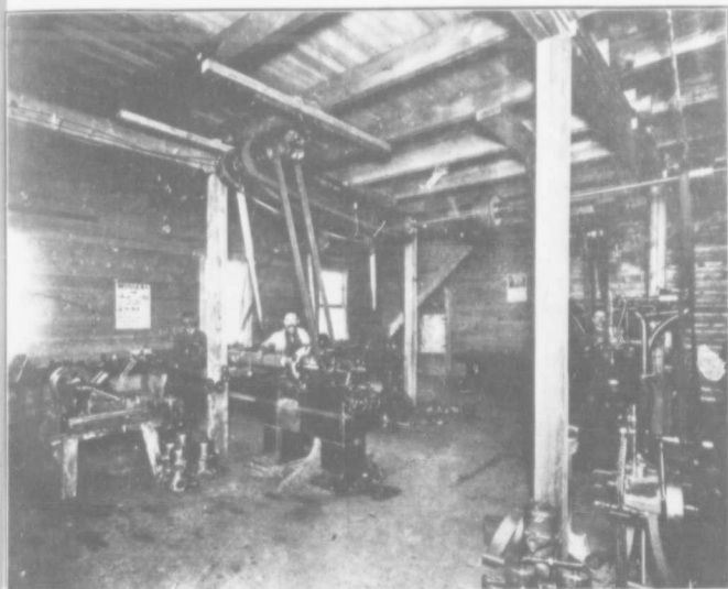
Inside View of a Section of the Plant.
