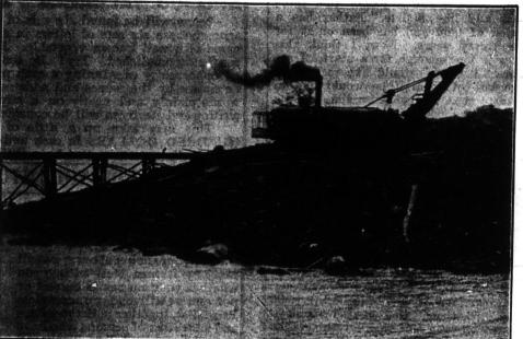
The only obstacle to a permanent roadway in the C.N.R. Rainy Lake district, now being replaced by a rock fill at cost of \$30,000,000.
