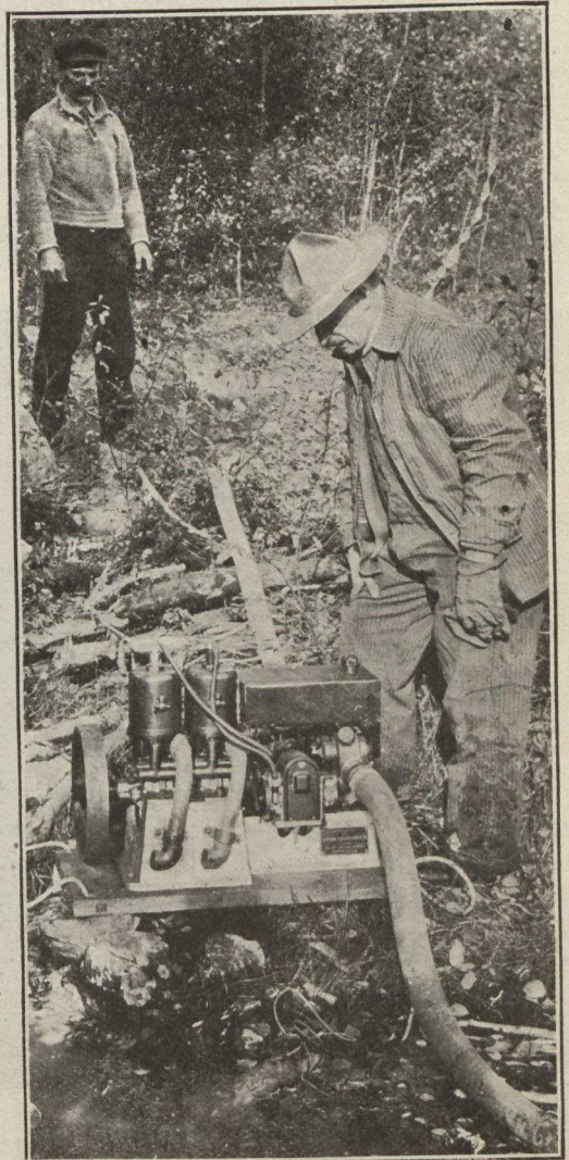
Pumping from a small creek in the Rocky Mountains Park.
