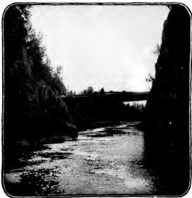
"THE NOTCH"—LOOKING DOWN.
