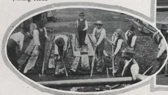
Laying Concrete Pavement
