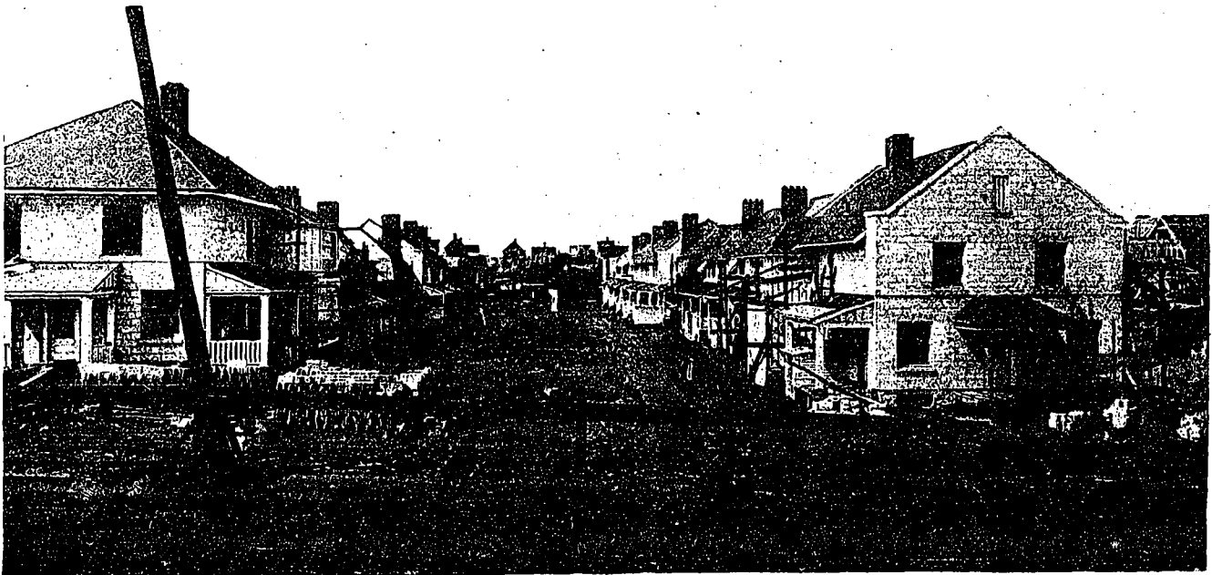
COURT SCHEME NEARING COMPLETION, RE-HOUSING DEVELOPMENT, HALIFAX, N. S.
