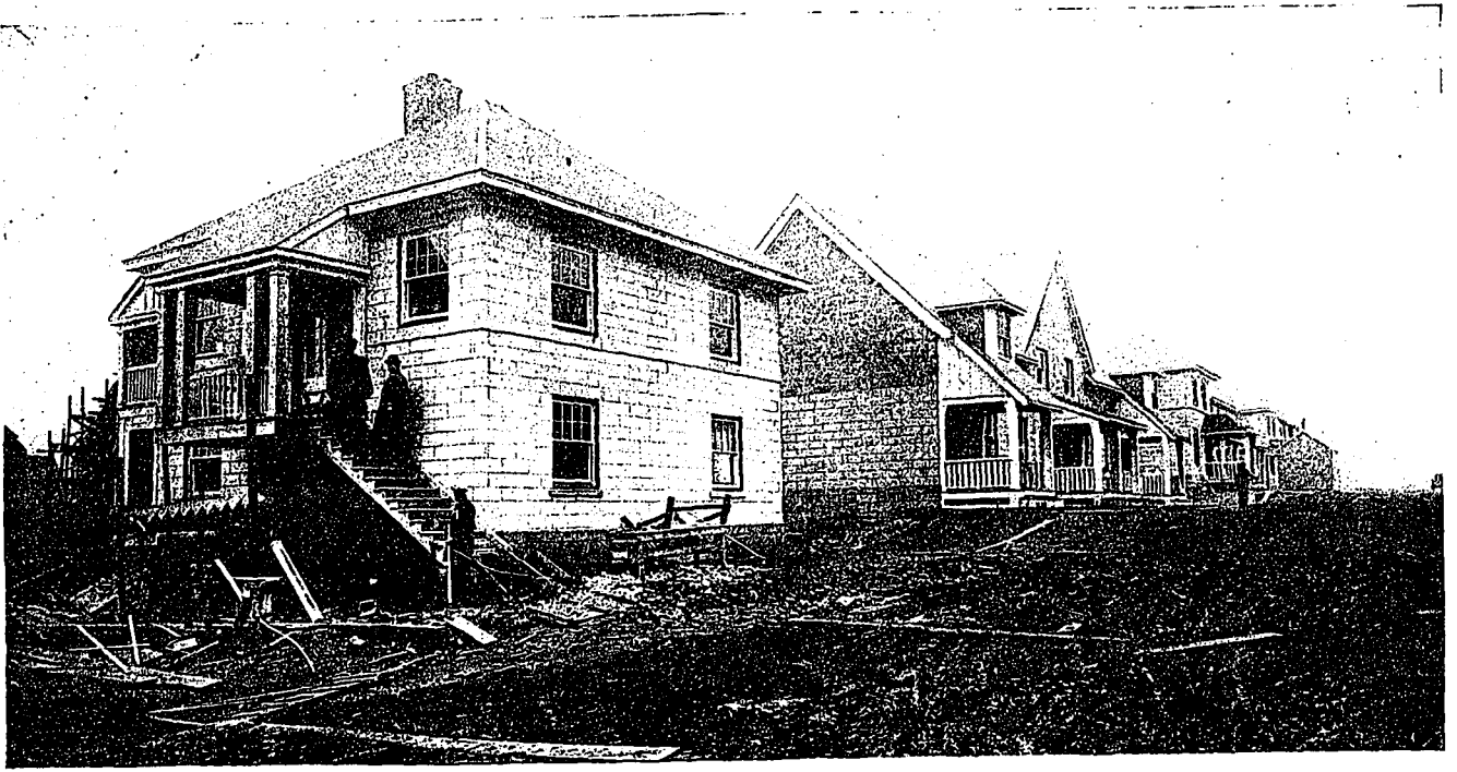
ROW OF HYDRO-STONE HOUSES WITH DWELLING CONTAINING TWO FOUR-ROOM APARTMENTS IN FOREGROUND, RE-HOUSING DEVELOPMENT, HALIFAX, N. S.
