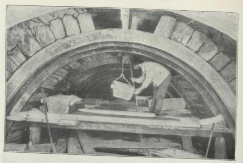
MASONRY ARCHING IN TUNNEL.
