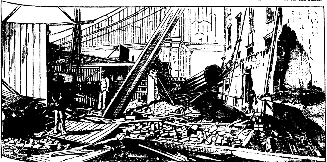
FIG. 1.—POSITION OF THE THREE BOILERS AFTER THE EXPLOSION.
