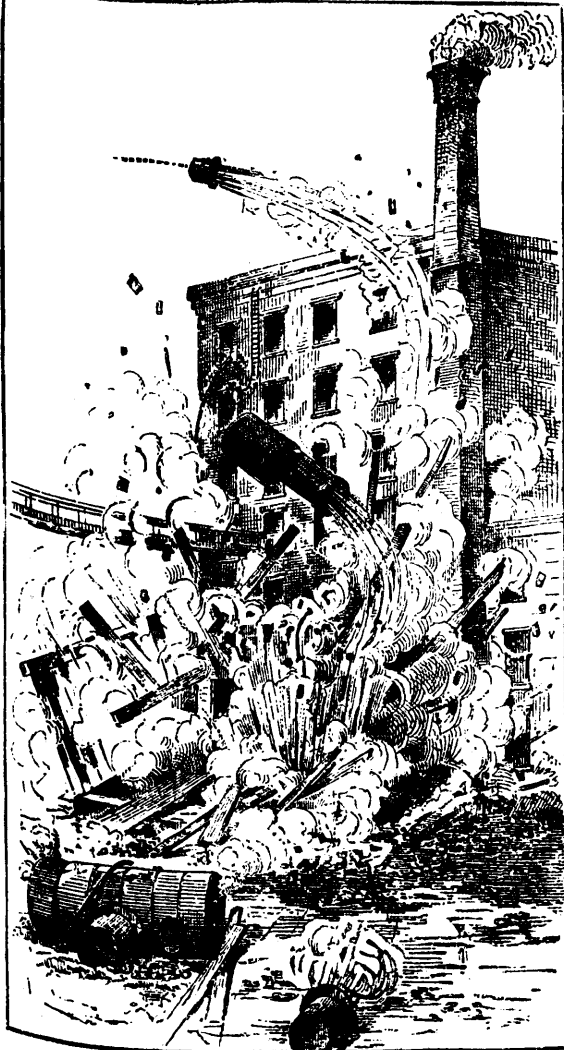
FIG. 4.—EXPLOSION OF THE BOILERS.
