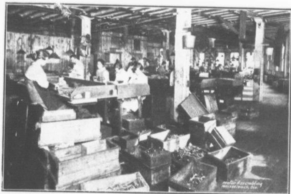
Showing a section of the factory where Meisselach motors are being assembled.
