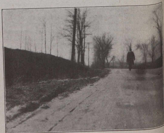
Fig. 3.—Break in Plainfield Road.
