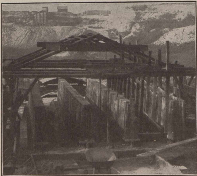
Fig. 8.—Grit Chambers Under Construction—Showing Formwork, Etc., and General Method.
