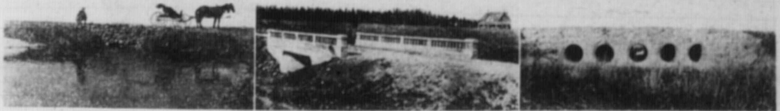
Some of the Bridges and Culverts that Wallace is Building for Prosperity. These Structures will be giving service when the History of the Millennium is being Written. Double 24 inch Pipe Culvert at Capacity A 14 foot Bridge with Macadam Concrete Railing A Battery of Five 24 inch Pipes Set in Concrete
