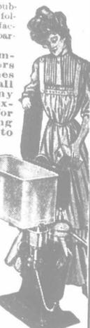
To oil the Dairy Tubular, pour a spoonful of oil into the gear case once or twice a week. Self oiling. No oil cups, tubes or holes.
