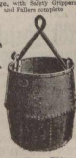
42—Mining Ribble with or without Valve in bottom
