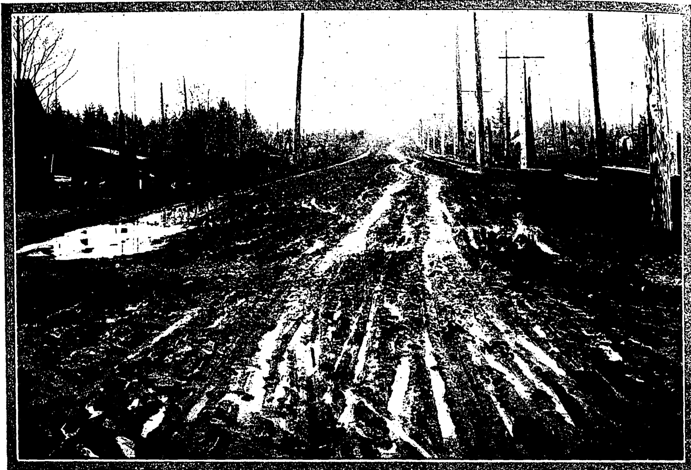
Photo by courtesy of the Columbia Bitulithic Company
