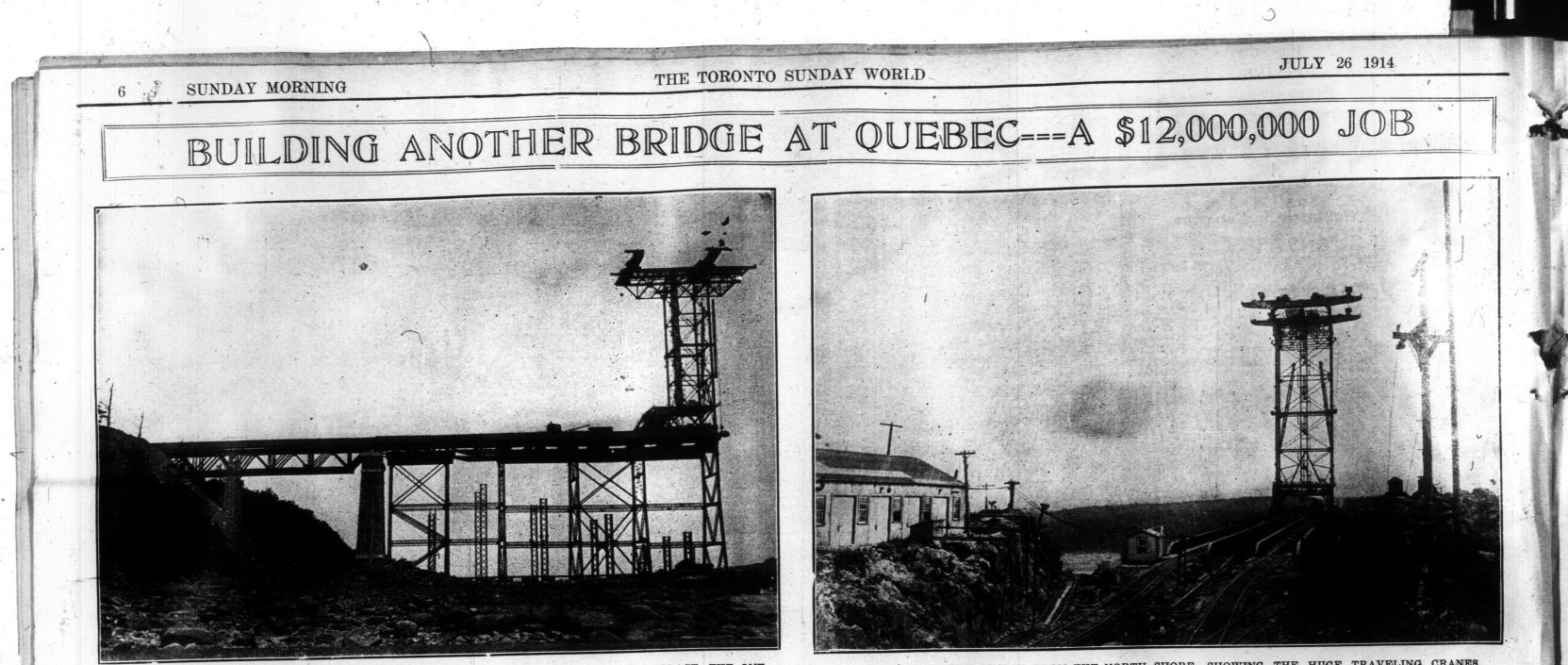
THE TEST COMPLETED SECTION OF THE NEW QUEBEC BRIDGE, WHICH IS TO REPLACE THE ONE THAT COLLAPSED SEVERAL YEARS AGO. THE APPROACH TO THE BRIDGE FROM THE NORTH SHORE, SHOWING THE HUGE TRAVELING CRANES, WEIGHING A THOUSAND TONS. AND WHICH ARE 358 FEET ABOVE WATER.
