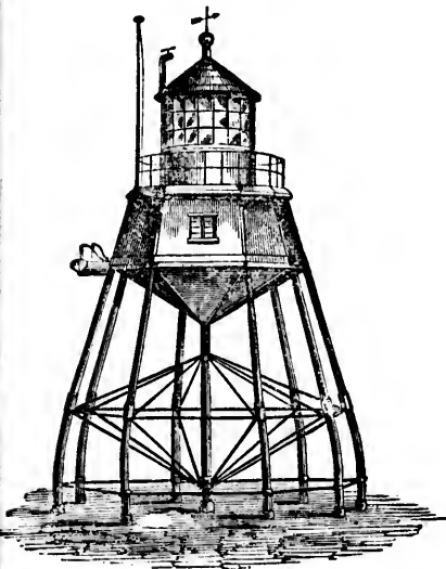
The Maplin Lighthouse, erected by Mr. Walker, upon Mitchell's screw-pile foundation.
