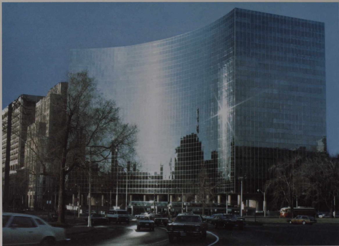
Hydro Place, headquarters of Ontario Hydro, was the first northern office building in the world built without a furnace. The heat generated by people and machines warms and cools the building.
