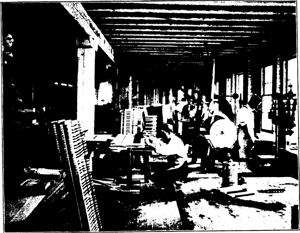
Another Part of Key Room.
