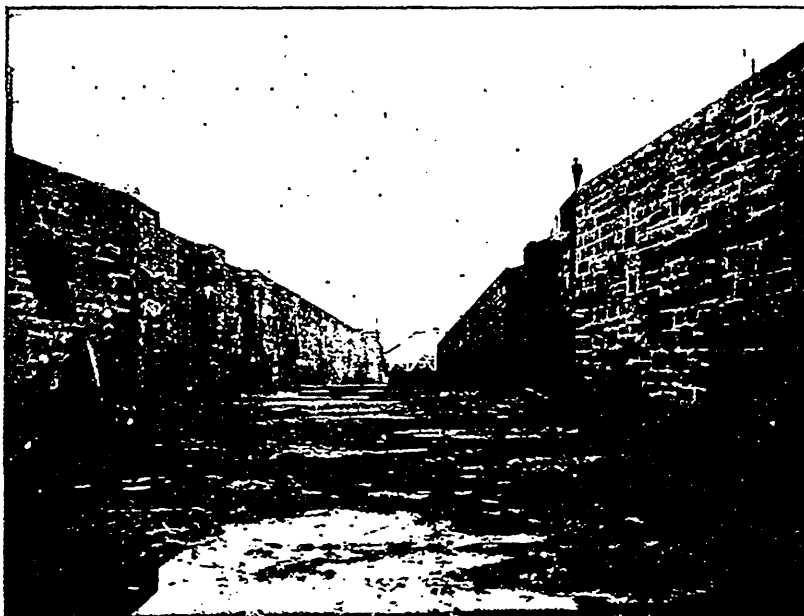
WEST END APPROACH, SHIP CANAL, BEFORE COMPLETION.
