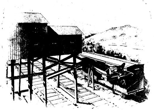
For loading Coal or Ore in Box Cars.
