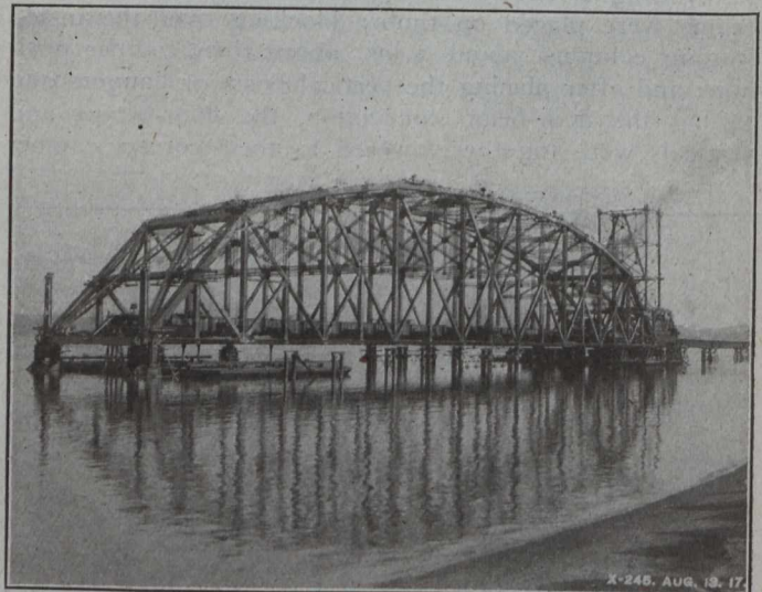
Fig. 10.—Suspended Span Erected at Sillery Cove
