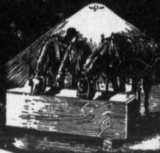
Pumps the Water
