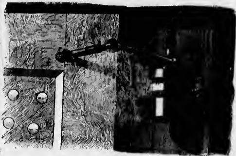
Check on Jamb, Door open.
